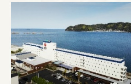
Ooedo-Onsen Monogatari Nanki Kushimoto (Higashi Muro County, Wakayama Prefecture)
