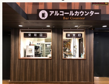
Installation of a counter for alcoholic drinks (Kinugawa Kanko Hotel)
